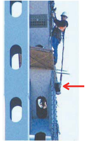
Figure 1. An example of an anchor point located below the worker's feet.
