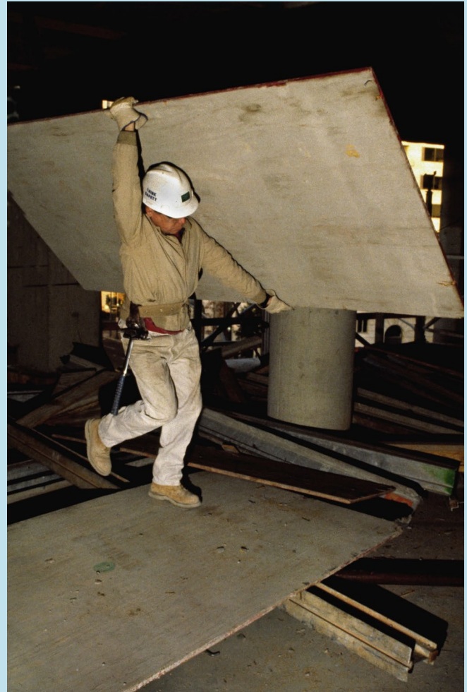
Drywall manual handling risk factors: weight, handling ease and awkward postures.
