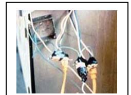
Improper Wiring
